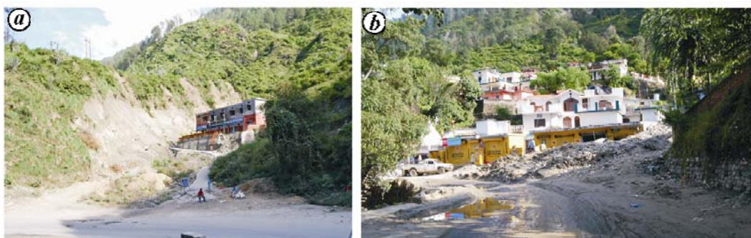
Figure 5. a , Disaster in the making – defying all safety norms, a school was allowed to be constructed on old landslide debris on the bank of a seasonal stream. b , Shops and houses constructed along the bank of an ephemeral nala. Shops seen buried under debris from upslope due to heavy rain in September 2010.
