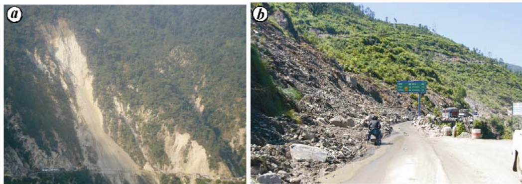
Figure 4. a , Kaliyasaur landslide (along NH-58) reactivated due to heavy rainfall in September 2010. It has become a major bottleneck for vehicular traffic on the Rishikesh–Badrinath road. b , Road widening work in progress along NH-58. Note the massive debris that has slid down after the angle of repose was disturbed during road-widening work followed by heavy precipitation in September 2010 along NH-58.
