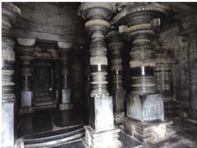
**Figure 3.** An interior view of the Parshvanatha Temple (Jain Basti; see Figure 1 for location) constructed from the stones (chlorite schist) mined from the nearby quarries.
