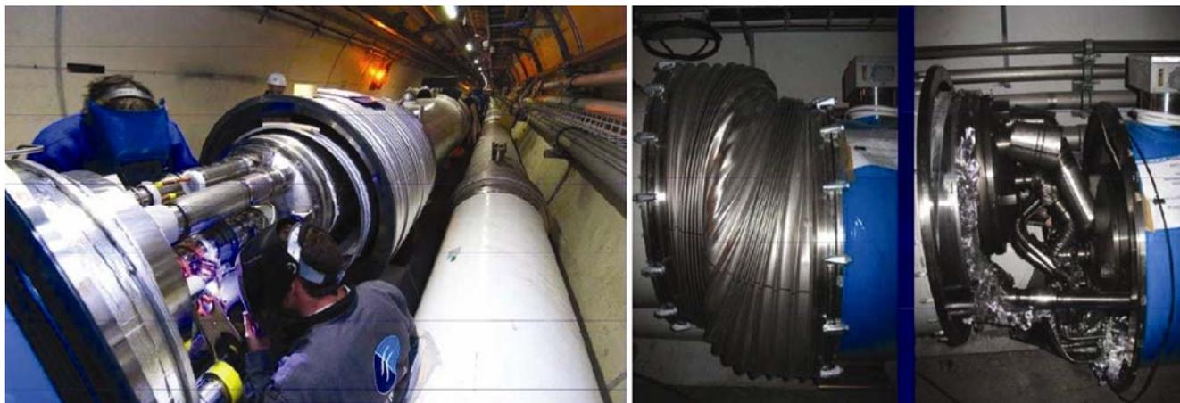
**Figure 4.** The quadrupole–dipole connection: undamaged (left panel) and damaged (right panel).
