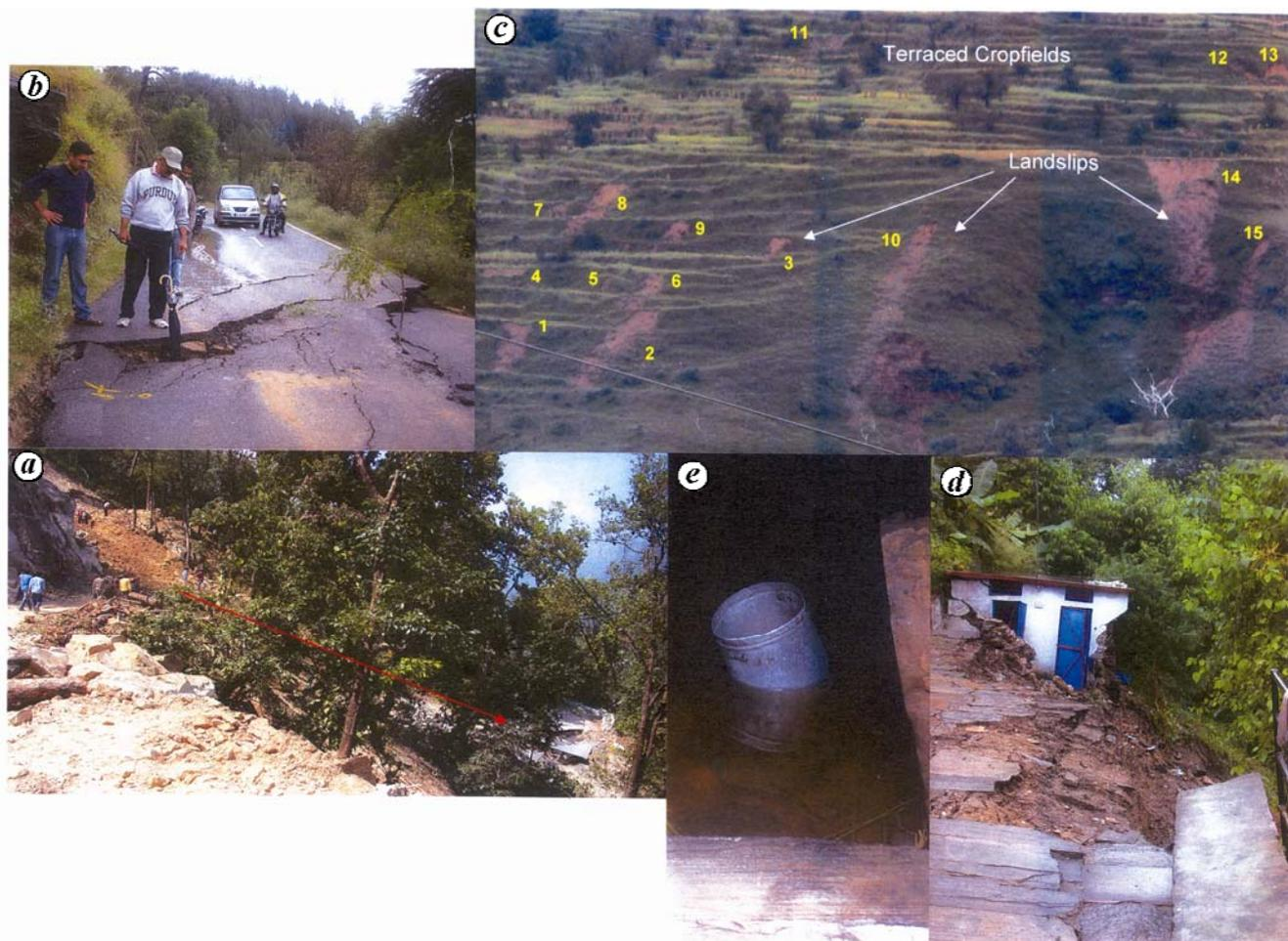
**Figure 1.** Damages due to catastrophic event. *a*, Huge mass of landslide which took a piece of the National Highway 87 nearly 30 m downslope in Nainital District. *b*, Sinking of National Highway 87 in Almora District. *c*, Numerous newly developed landslips of different sizes. *d*, Damage to building. *e*, Water-filled ground floor of a cattle shed in a rural building.
