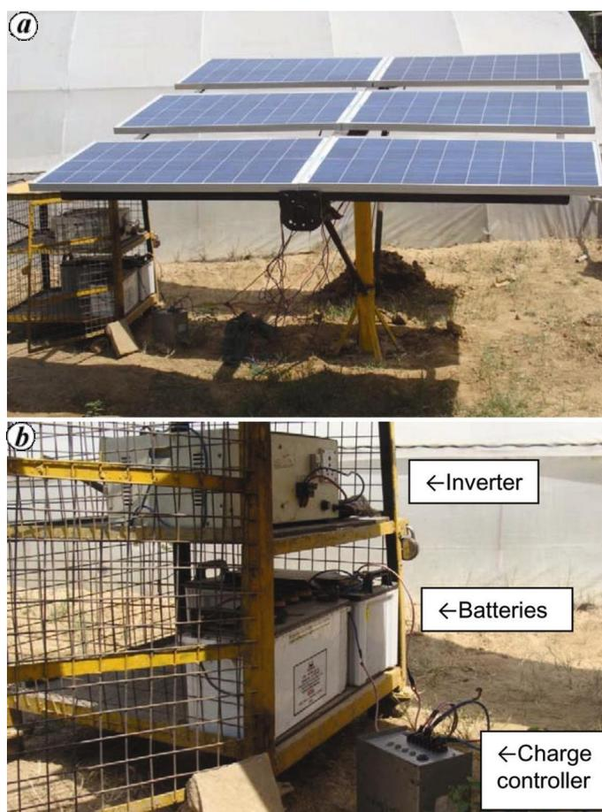
**Figure 1.** a, Solar modules of 600 W power pack system. b, View of inverter and batteries.
