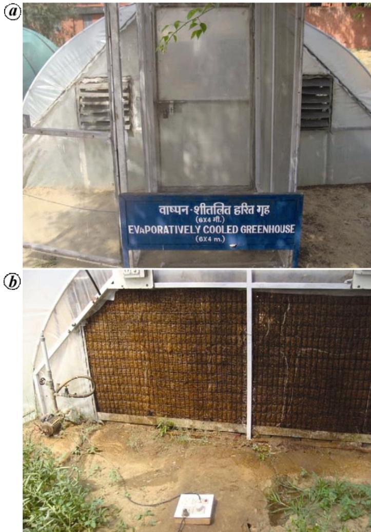
Figure 2. Solar photovoltaic-powered exhaust fans (a) and fan-pad cooling system (b) in the greenhouse.
